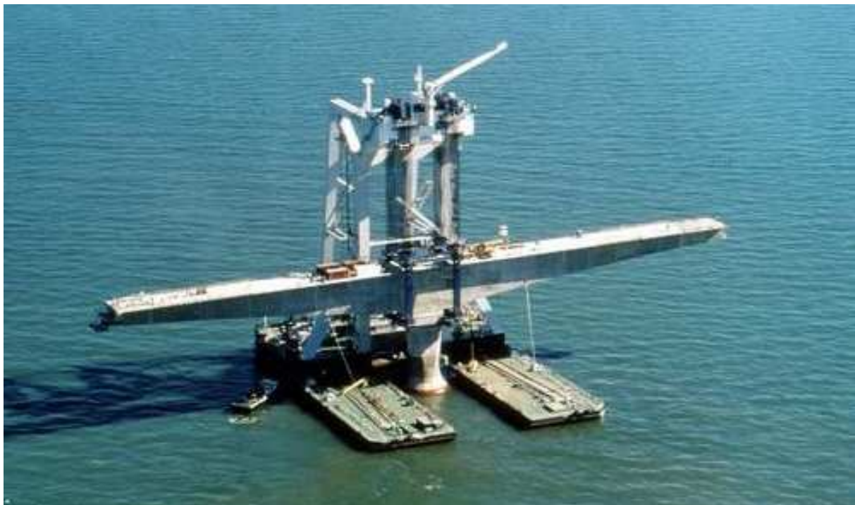
Figure 5 : Placing of a main girder
