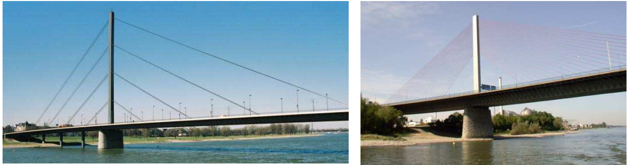
Figure 8: From few to many cables – Oberkassel Bridge (left) & Bonn-North Bridge (right)
