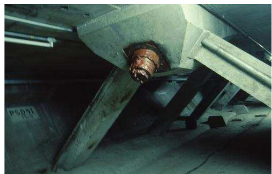
Figure 11 : PT tendons equilibrating tension in the struts
