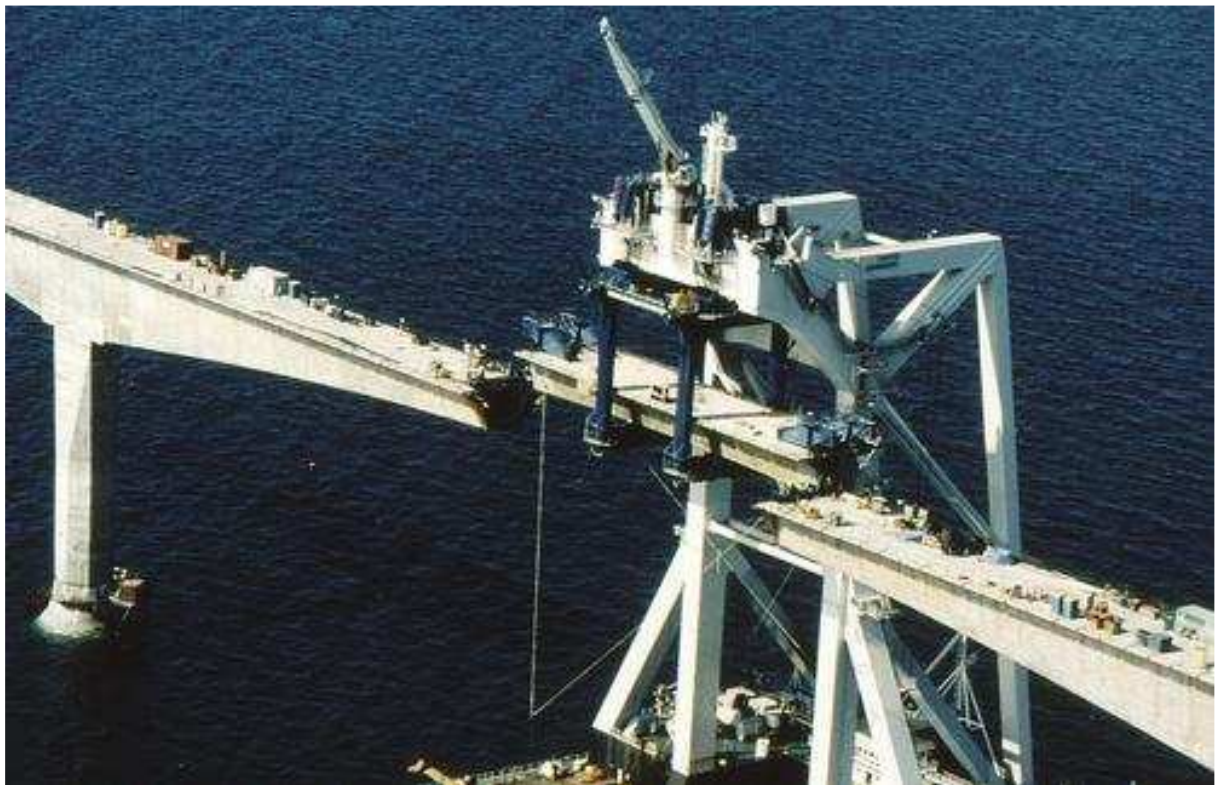
Figure 6 : Drop-in-Span installation
