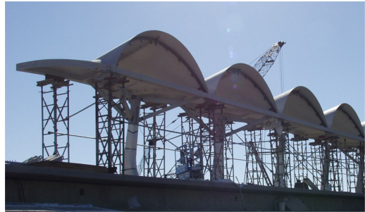
Figure 5. Canopy construction with temporary scaffolding (Adeeb et al., 2005).
