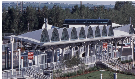
Figure 6. The LRT Station. (Lafarge Canada Inc.).
