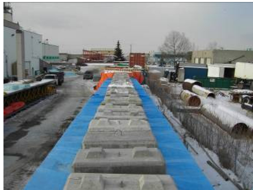
Figure 10. The bridge full-scale test.
