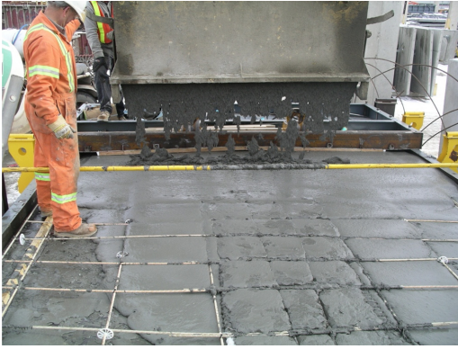
Figure 11. Casting of the girder nearing completion.
